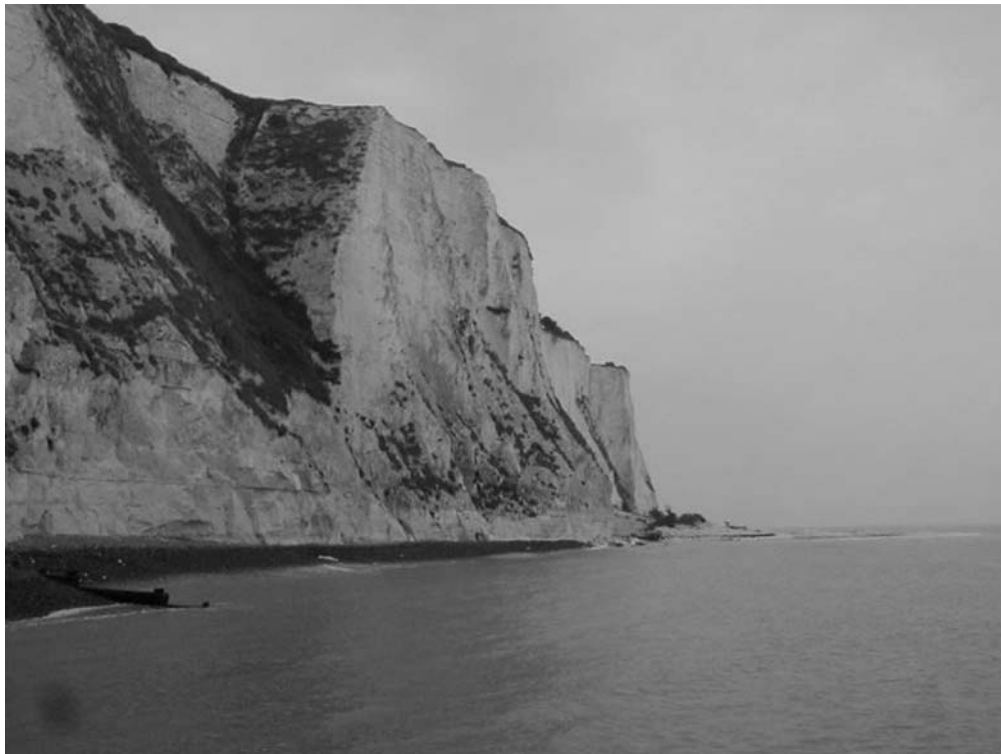
Figure 4.23: View looking north of St Margaret's Bay, Kingsdown to Dover GCR site. (A) Small, fringing beach of flint, mostly derived from recent cliff falls; movement alongshore is restricted by fall debris; (B) large toe of a slide extending beyond low-water mark; (C) cliff being eroded where previous rock fall has been completely removed; (D) vegetated slope that developed behind a former slide toe and debris; these features then protected cliff-foot bedrock from erosion; (E) typical upper cliff profile above debris slopes. (Photo: V.J. May.)
