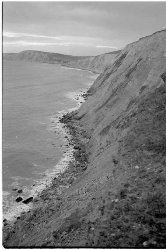
Figure 4.19: Characteristic slope failures at Compton Down, looking west, showing shallow slides in chalk rock. (Photo: V.J. May.)
