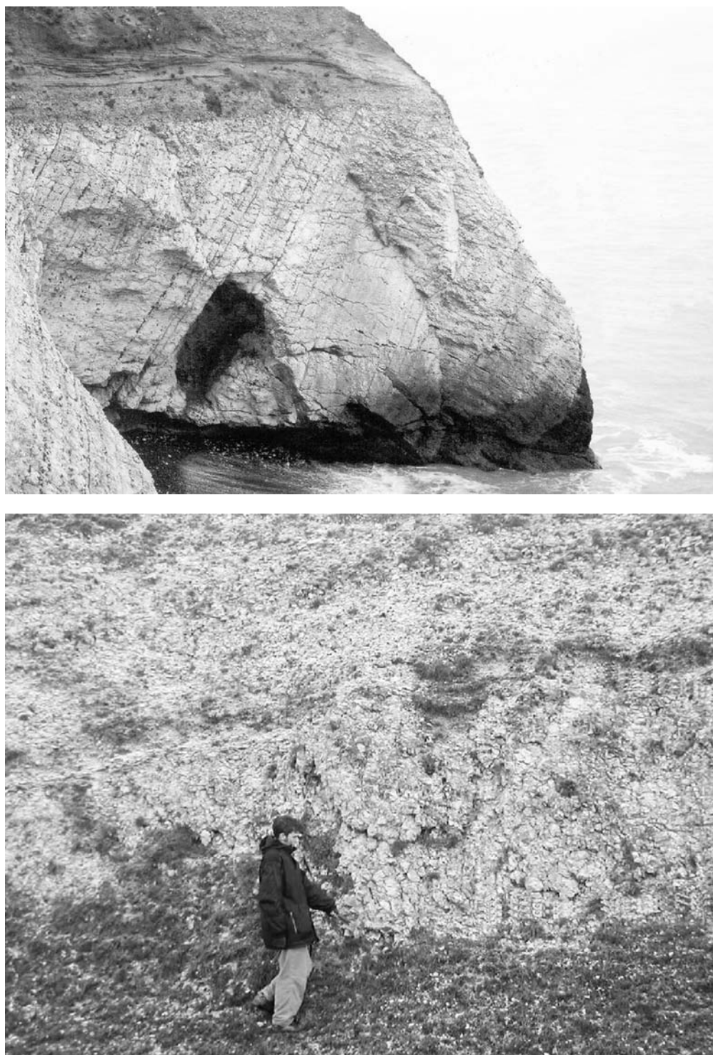
Figure 3.62: (a) Turonian–Coniacian Lewes Nodular Chalk Formation at the western end of the Compton Bay GCR site, adjacent to Freshwater Bay, Isle of Wight. (b) Base of the Lewes Nodular Chalk Formation in the Compton Down Military Road section in the Compton Bay GCR site, Isle of Wight. (Photos: R.N. Mortimore.)
