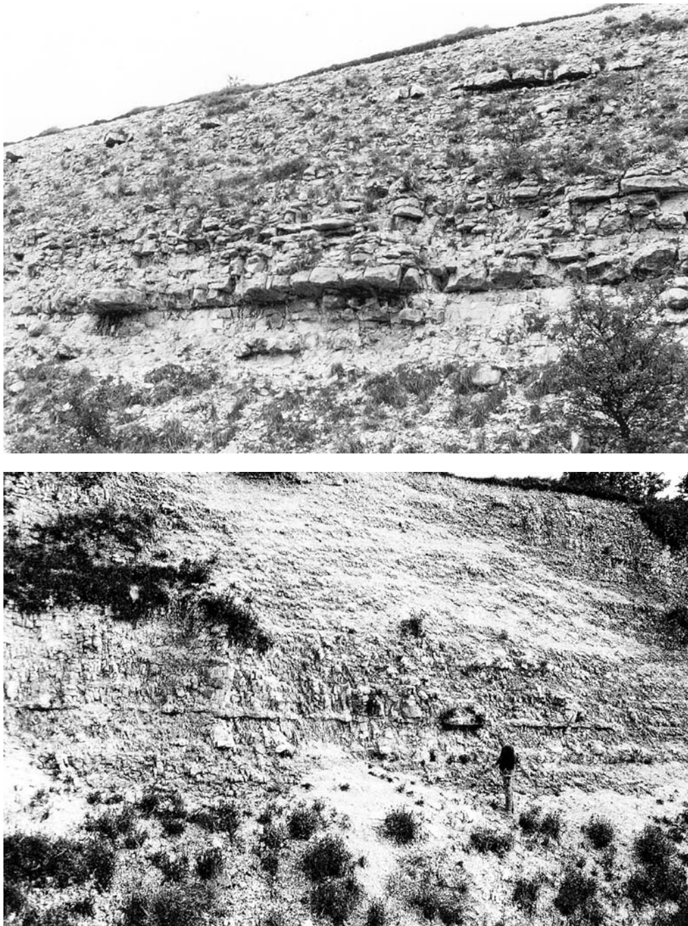
Figure 5.17: Enthorpe Railway Cutting in the highest Turonian and Lower Coniacian Burnham Chalk Formation. (a) North side of cutting looking NNW. (b) South side of cutting looking south-east. (Photos: C.J. Wood.)
