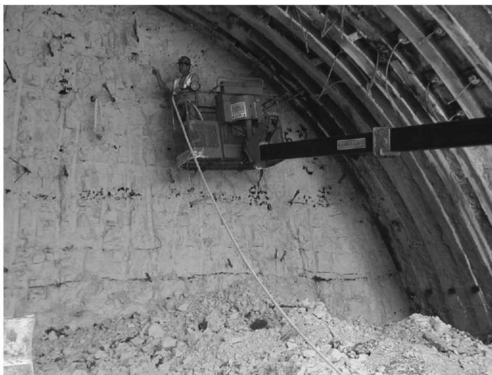
Figure 3.127: (a) The cliffs at Joss Bay, showing Whitakers 3-inch Flint Band (W3) and strongly cryoturbated chalk and flint. (b) Giant flint columns emanating from Bedwell's Columnar Flint Band, South Portal, Ramsgate Harbour Tunnel (arrowed). (Photos: R.N. Mortimore.)
